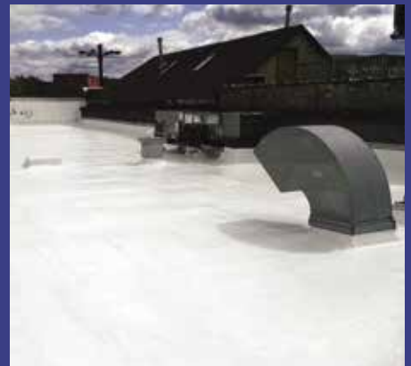
Liquid-Applied Roofing
