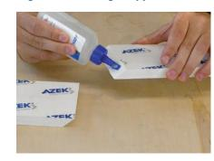
Use AZEK Cellular **PVC** Cement for securing joints and other trim connections requiring tight compression.
