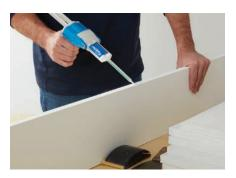
Use AZEK Fast Cure and Slow Cure to fill gaps and other trim connections that do not require tight compression. Use a putty knife to distribute and sand when dry for a smooth finish.
