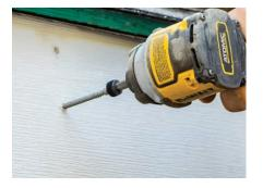
Drive fastener at 90° angle to preset level below trim surface.
