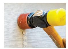
Place plug with trim surface side-up into hole. Gently tap plug until flush with the trim.
